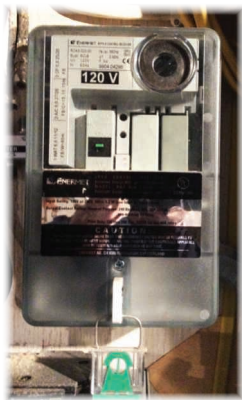
Example of a load management box
