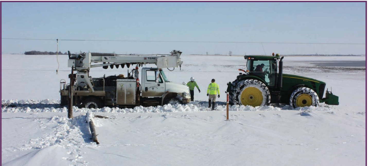
Charles Mix member Gary Hrdlicka offers extra horsepower to the Douglas Electric crew. Hrdlicka pulled the crew through deep snow in order to make line repairs.
