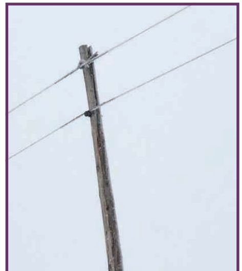
Ice weighed down the lines and split the top of this pole.
